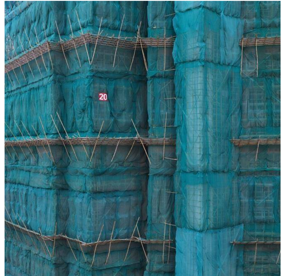
Toothpicks of bamboo scaffolding
